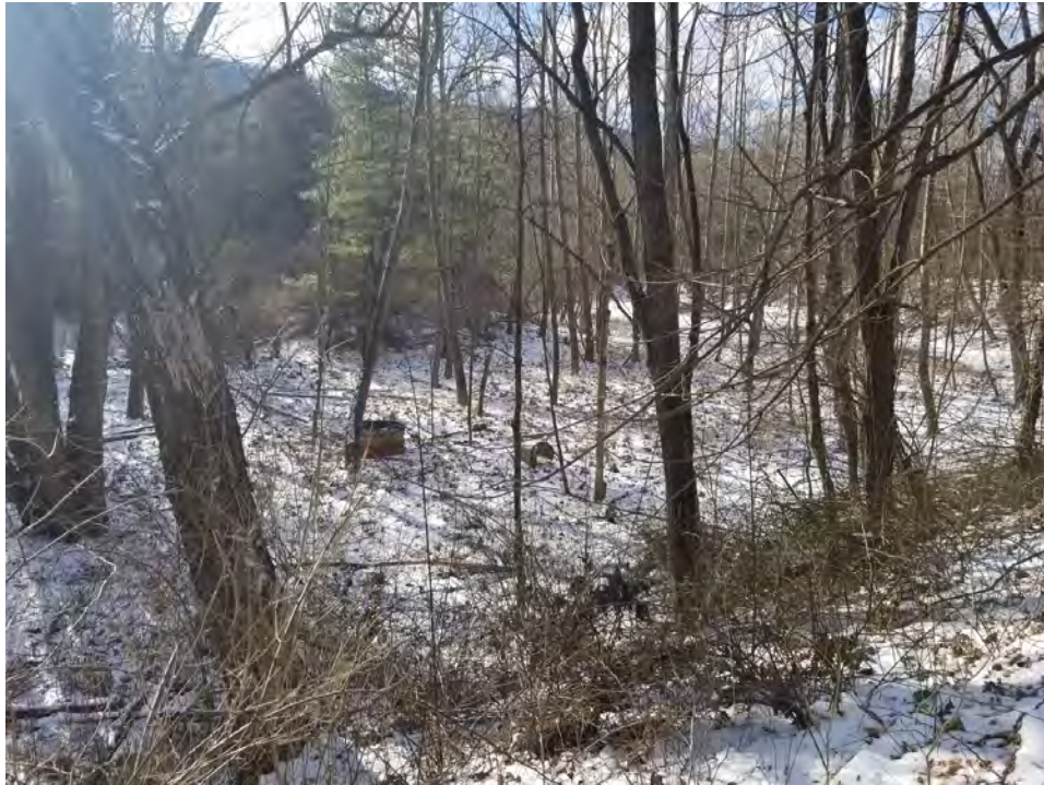
Photo 1: Riser structure in former Ash Disposal Basin (photo taken by GAI, dated 01/24/2025)
